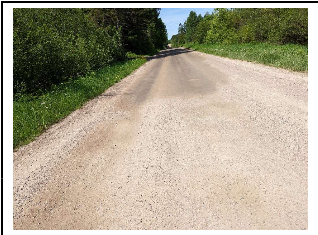
Photo 4 West approach from centre of structure
