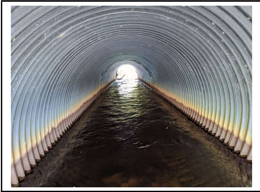
Photo 7 Typical view of east interior barrel looking south
