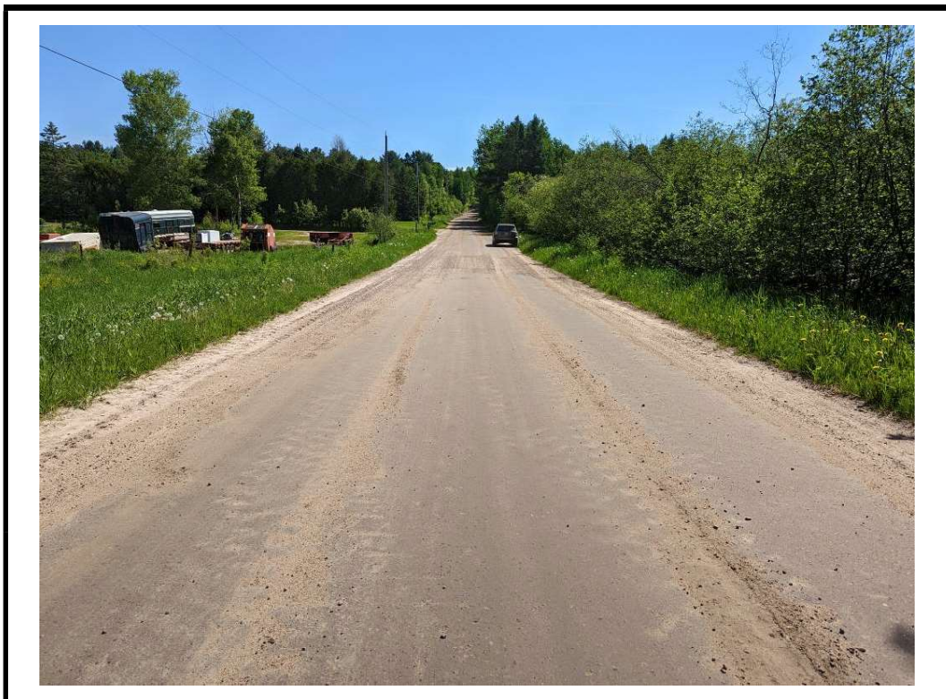
Photo 2 Structure from west approach
