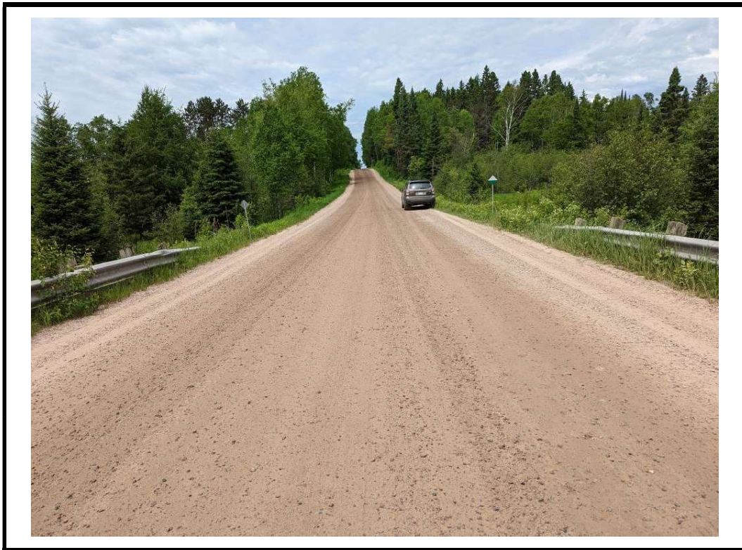
Photo 3 North approach from centre of structure
