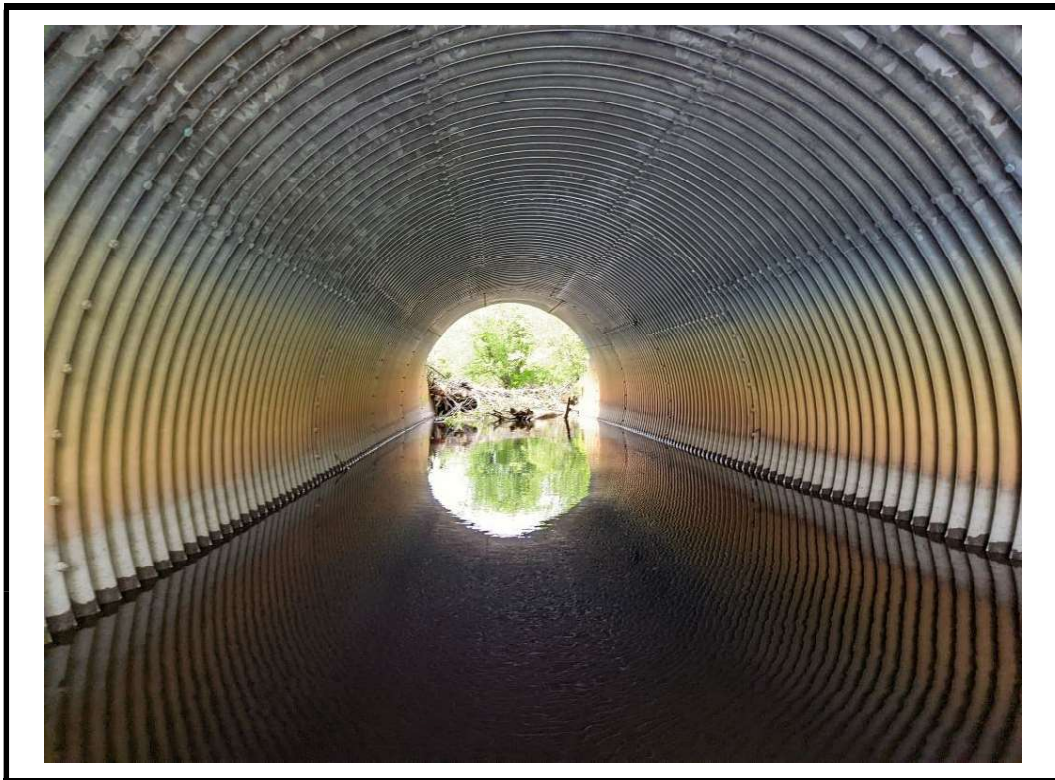
Photo 11 Typical view of south culvert barrel looking west
