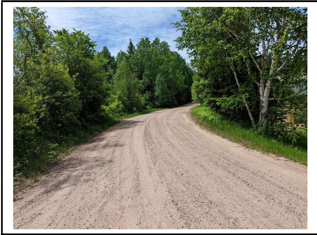
Photo 1 Structure from east approach
