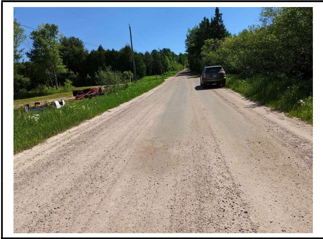
Photo 3 East approach from centre of structure
