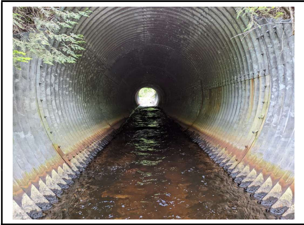
Photo 9 Typical view of interior barrel looking south
