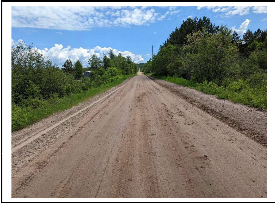
Photo 3 East approach from centre of structure
