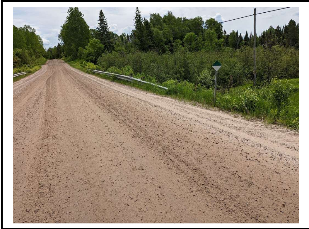
Photo 9 Gravel approach wearing surface
