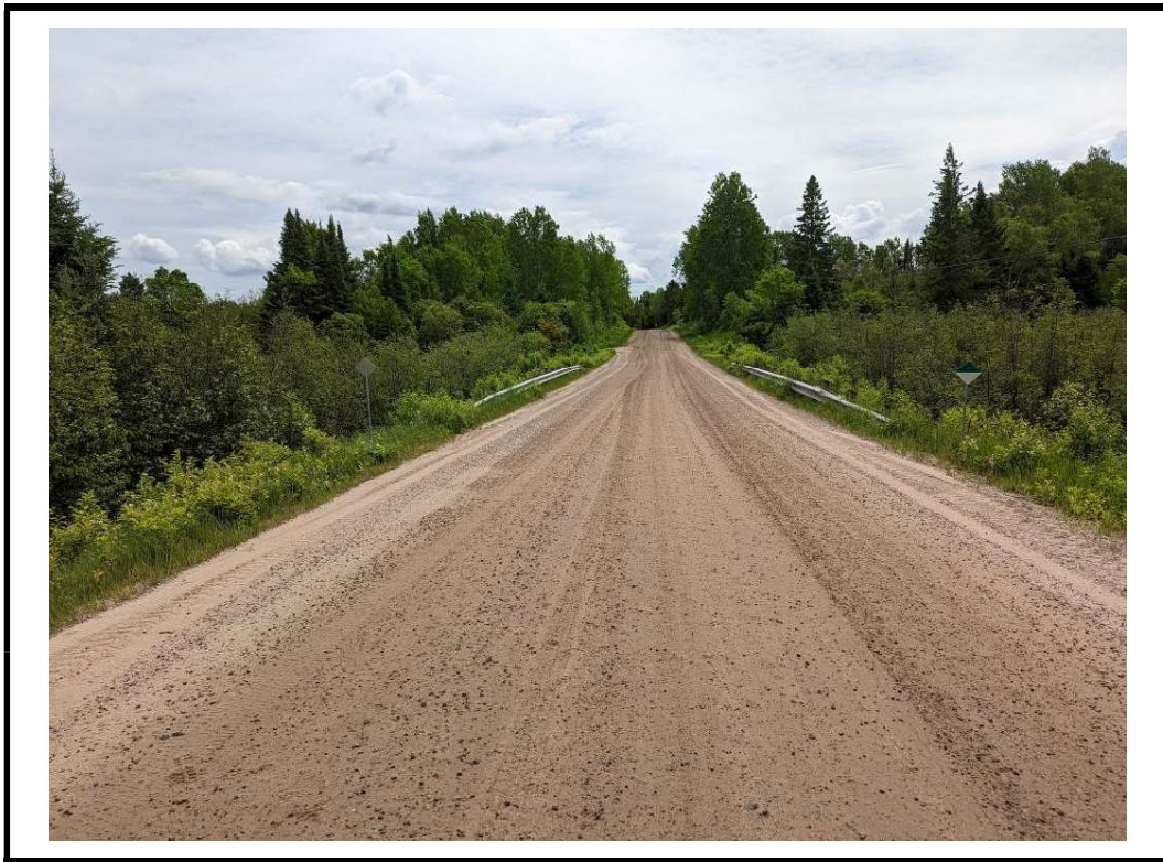
Photo 1 Structure from north approach
