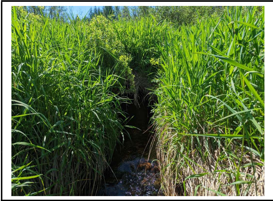
Photo 5 Heavy vegetation grown at north side of barrel
